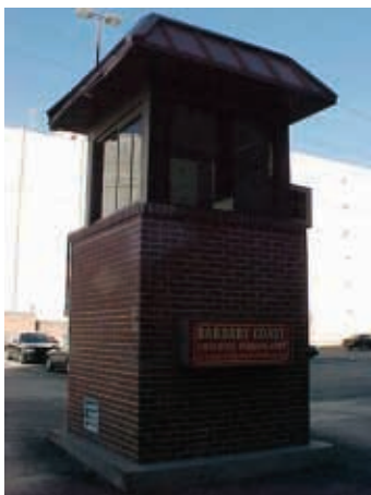
The security tower for the employee parking area off of Flamingo. I always got a kick out of the way it resembled a prison guard tower.
