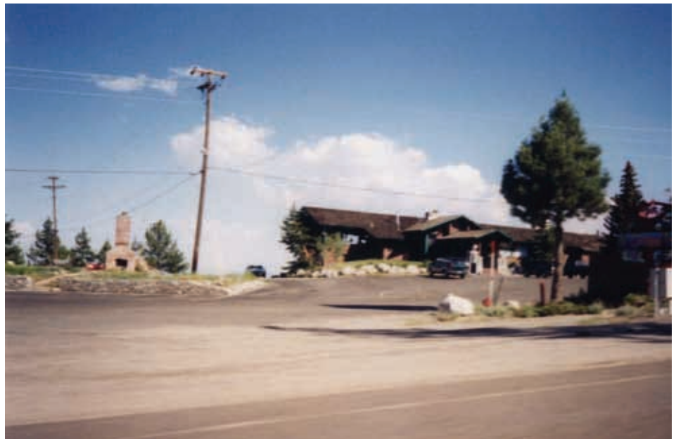
The fireplace from the original building sits to the left of the new structure built in 1965
