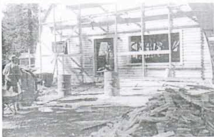
Quonset Hut becomes George's Gateway at South Lake Tahoe
