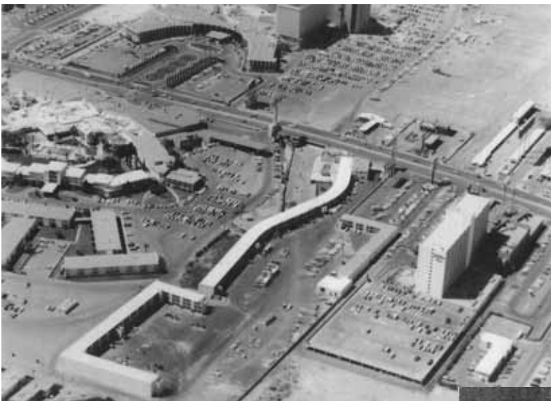
Aerial view of the Flamingo Capri with the new Imperial Palace East building
