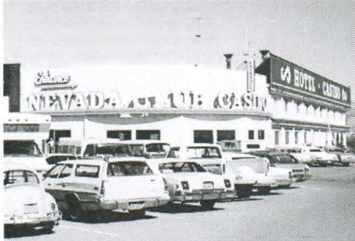
The Nevada Club probably sometime after 1975 showing some additions and improvements.
