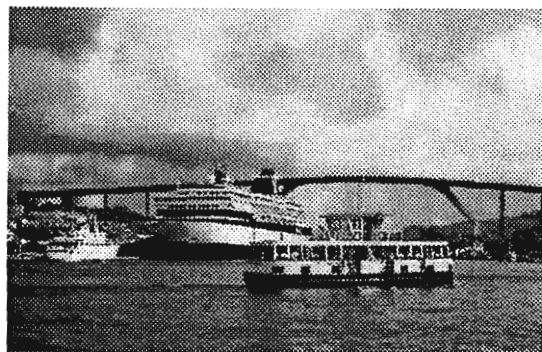
Queen Juliana Bridge with a ferry crossing the bay.
