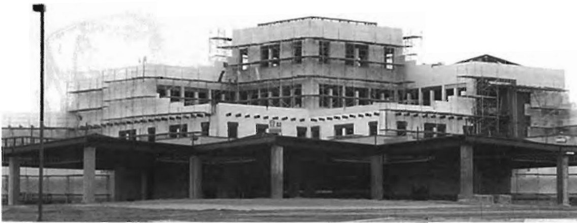
The walls go up on the new Isleta Casino
