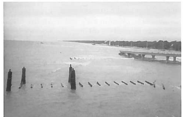
Water meets the dock and roadway
