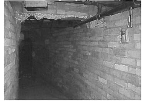
Tunnel between cabin 5 and cabin 3.
