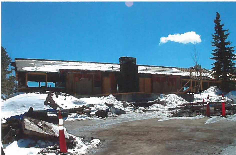
Construction on the Christmas Tree to produce The Tannenbaum.
