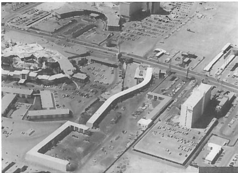
Aerial view of the Flamingo Capri with the new Imperial Palace East building
