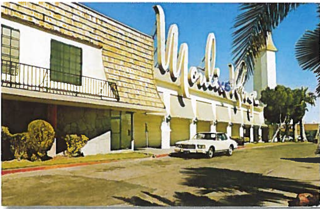
Changes implemented by Preddy including awnings and a shingled roof to the existing tower.
