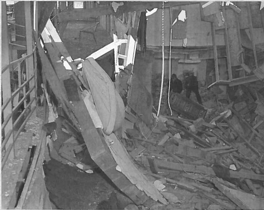
Investigators can be seen combing through the debris of the Orbit Inn hotel on January 7, 1967. Photo by Ken Jones.
