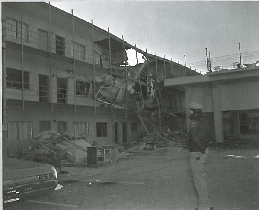
A view of the destruction from the parking lot. Photo by Ken Jones.
