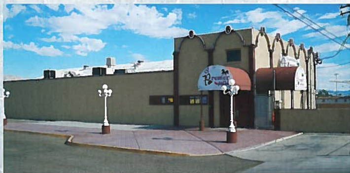
The Nashville Nevada building in its current state.
