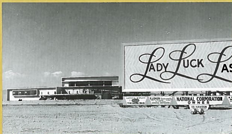
Construction photos of the Hacienda which was then going by the name of "Lady Luck"
